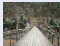
Yunnan suspension bridge, Shangri-La China
